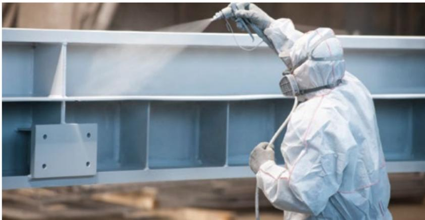
The **airless spraying method**, on the other hand, generates under high pressure a fine atomisation or a fine, airless atomisation of the fire protection coating that is applied as a high speed jet to the workpiece for the optimal surface look. The fire protection coating should first be applied after all steel components have been assembled and the roof rendered tight, but before building facilities obstruct access.
