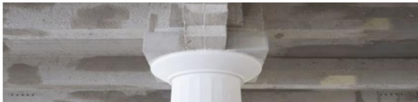
For renovation in areas with a fire protection requirement and high humidity, such as in swimming pools, or with high emission levels, such as in underground car parks / multi-storey car parks, the water pressure and weather resistant concrete fire protection coating **HENSOMASTIK® B 3000** is used. It improves the fire resistance duration of concrete and reinforced concrete components up to 120 minutes.
