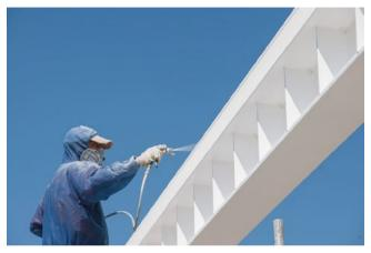
The application of 1C steel fire protection systems is usually carried out directly on the construction site. Water- or solvent-based intumescent coatings are used in particular for conversion and/or renovation measures in existing buildings.
