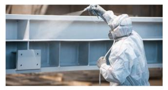
The **airless spraying method**, on the other hand, generates under high pressure a fine atomisation or a fine, airless atomisation of the fire protection coating that is applied as a high speed jet to the workpiece for the optimal surface look. The fire protection coating should first be applied after all steel components have been assembled and the roof rendered tight, but before building facilities obstruct access.
