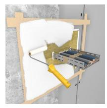
Apply **HENSOMASTIK<sup>®</sup> 5 KS Farbe/viskos** to cables and cable support structures (DFT  $\geq$  1 mm).
