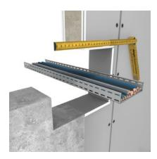
Measure length and width of the opening and penetrating services and transfer the sizes to the mineral fibre boards.
