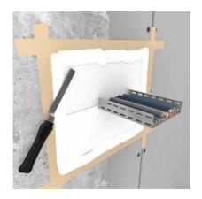
Smooth out the excess material with a spatula or putty knife to form the circumferential coating (DFT min. 1 mm).
