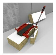
Cut the ready-to-use mineral fibre boards in perfectly fitting pieces to be installed precisely in the opening.
