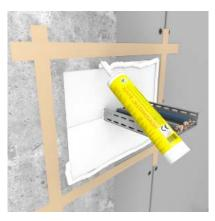
Apply a thick layer of **HENSOMASTIK® Acrylic** to seal the gap between mineral fibre boards and reveals.
