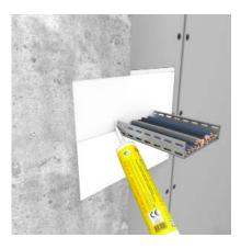
Fill all gaps > 10 mm with loose mineral fibre material, then with **HENSOMASTIK® Acrylic** from both sides in full depth.
